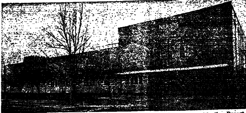
The former Aspro Nicholas research laboratories at Bath Road, Slough, now sold to Interdata, a mini-computer company and subsidiary of Perkin-Elmer Corporation. The price, say selling agents Jones Lang Wootton, was about £500,000. The property, built in 1969, originally contained research facilities and extensive
